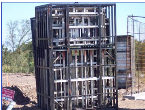
A Mercedes Homes metal-form panel awaits placement on a new home.
